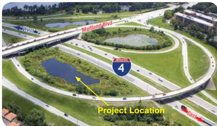
The Maitland interchange as it exists today
