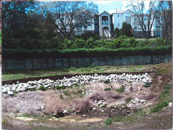
Fig. 31. (Before) Sinkhole that formed on June 11, 2002, in Pine Hills, Central Florida, and created a 150-ft-wide and 60-ft-deep cavity. It forced evacuation of 100 occupants living in apartments in background. (After) Site was permanently stabilized with a 50-ft-deep wall consisting of 3-ft-diameter interlocking piles.
